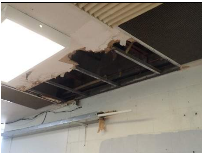
Damaged ceiling drywall in maintenance room
