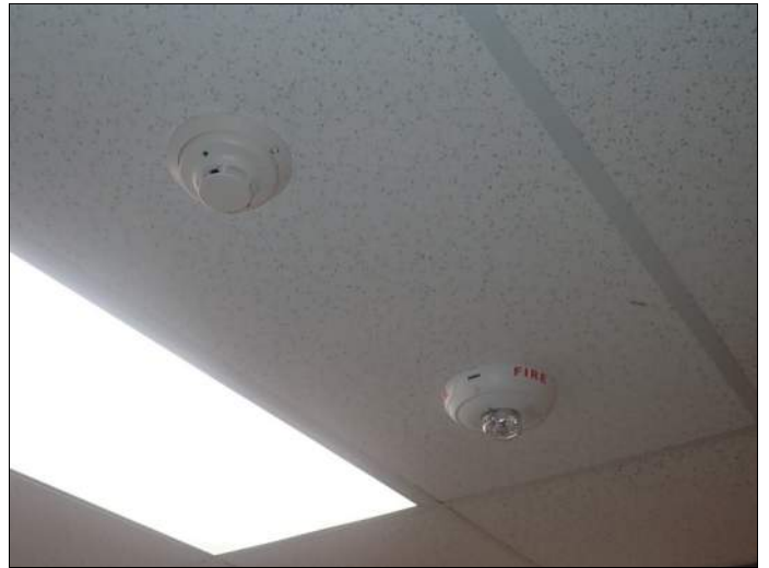
Typical audio visual alarm and smoke detector
