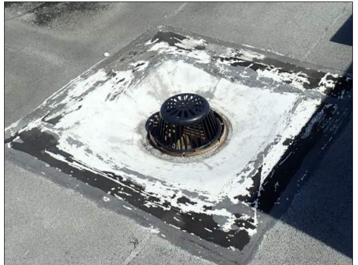
Typical internal drains on upper roof
