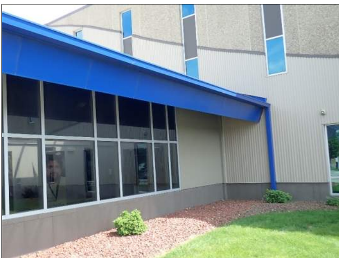
Gutter and downspout from metal panel roof
