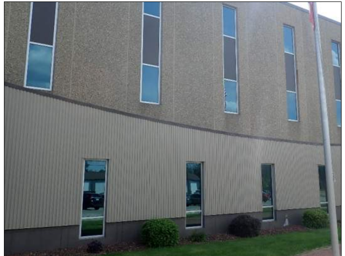
Exterior metal panel wall finish
