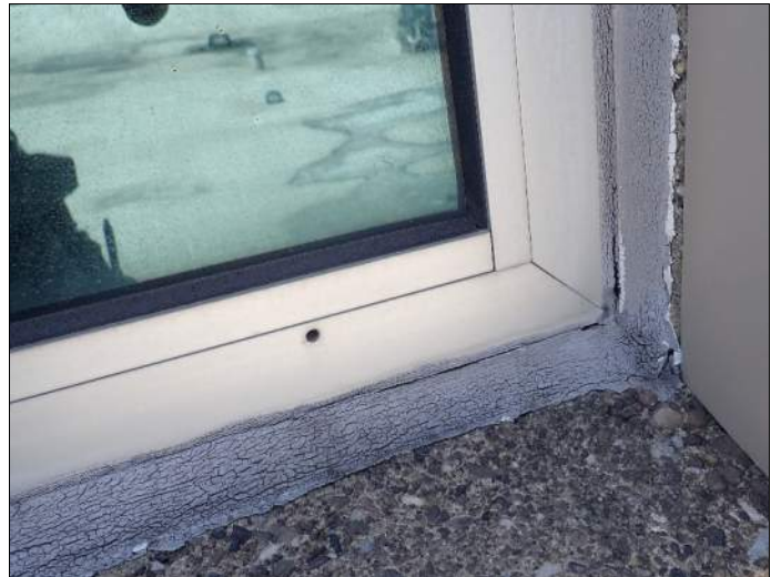
Deteriorating window sealant
