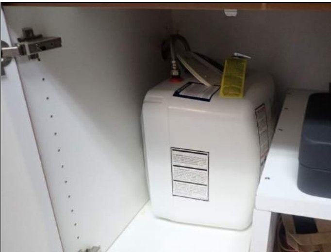
Water heater beneath sink
