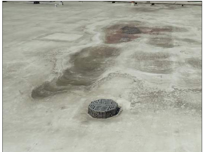
Typical internal drain on lower roof
