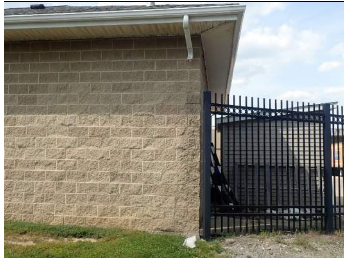
Disconnected garage downspout
