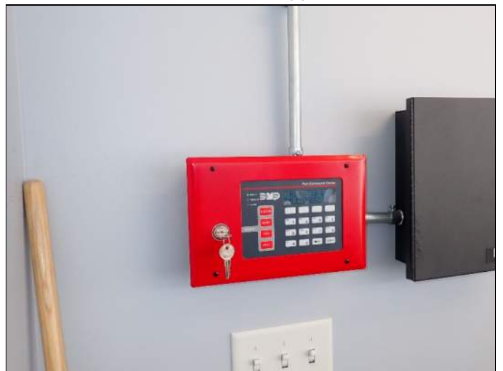
Fire alarm system secondary controls
