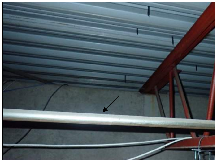
Typical water distribution tubing
