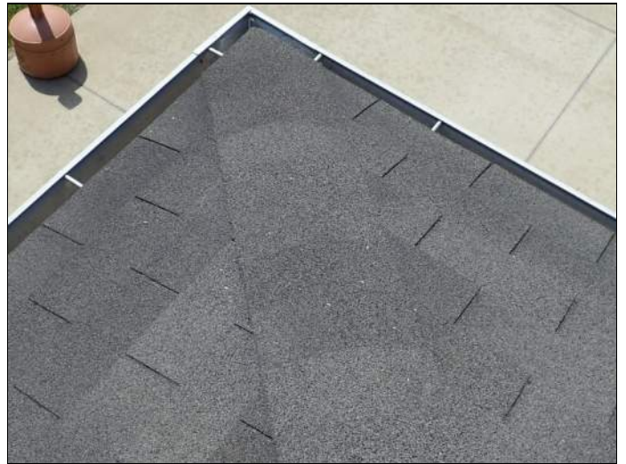
Typical shingles on hip roof
