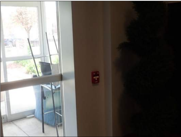
Typical fire alarm pull station
