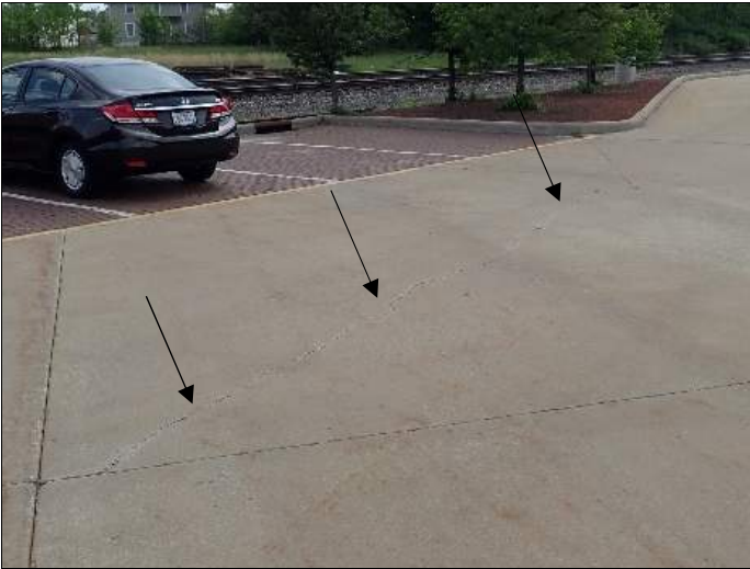
Typical shrinkage crack in concrete
