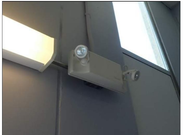
Typical emergency light fixture
