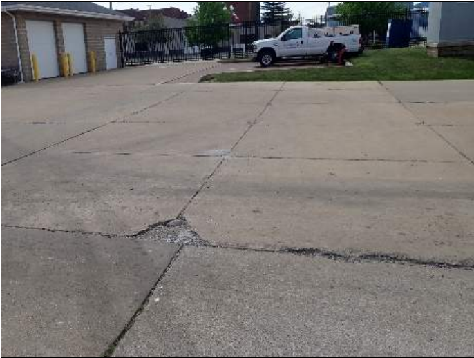
Typical deterioration of rear parking area concrete
