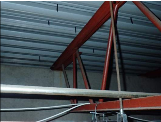
Steel joist bearing on precast concrete wall panel
