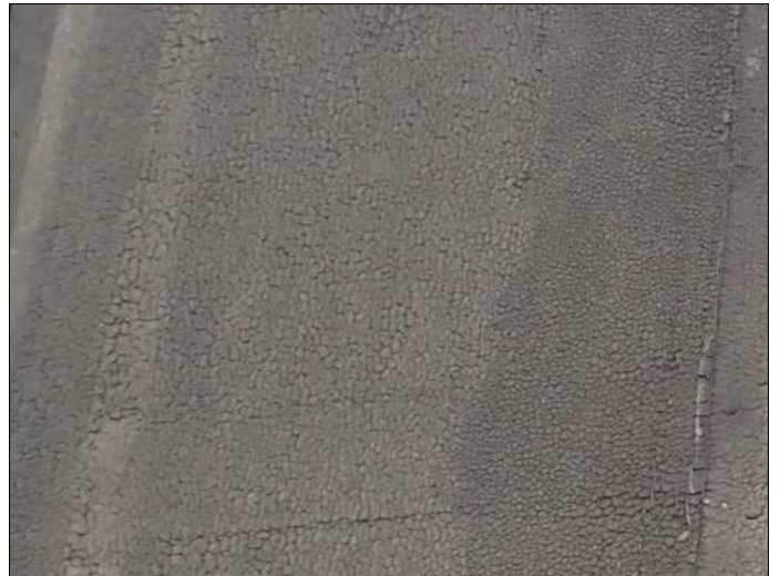
Typical alligator cracking of roll roofing
