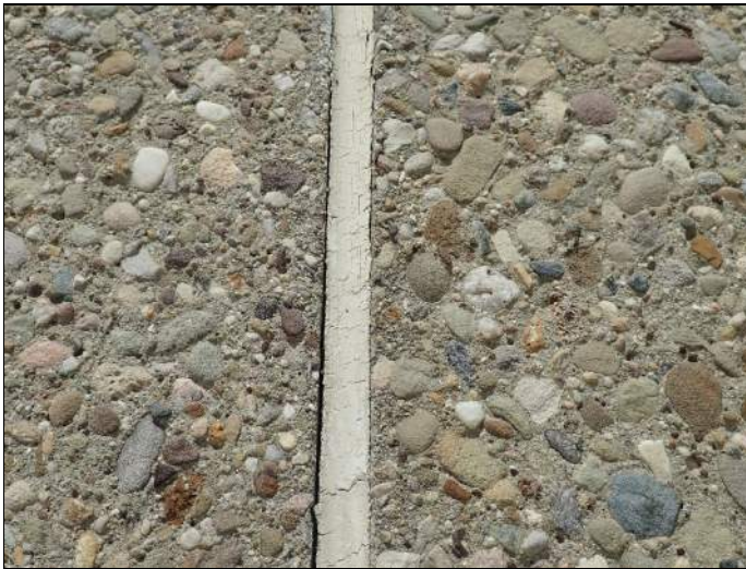
Deteriorating sealant at wall panel construction joint
