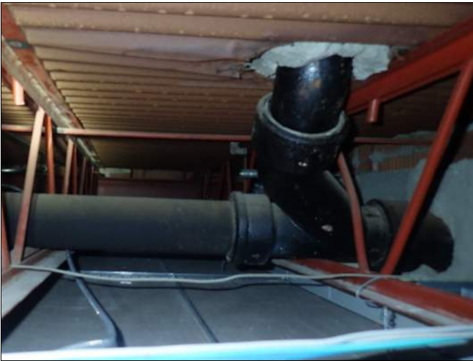
Typical sanitary waste tubing
