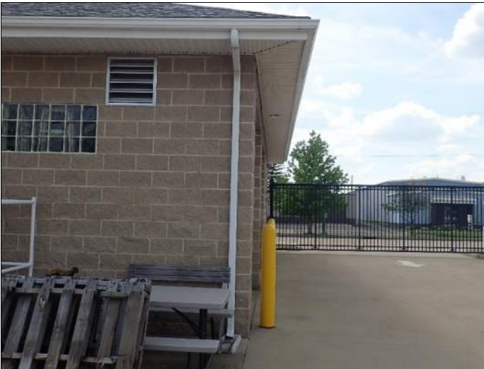
Typical garage gutter and downspout
