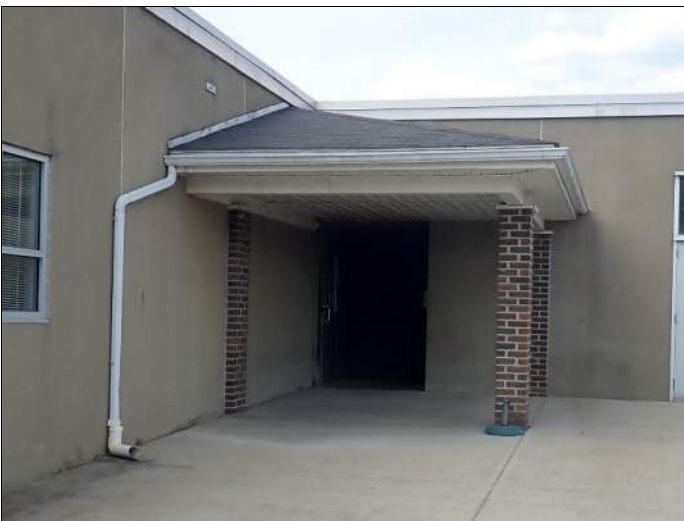
Hip roof gutter and downspout
