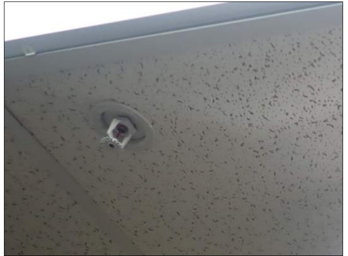
Typical sprinkler head
