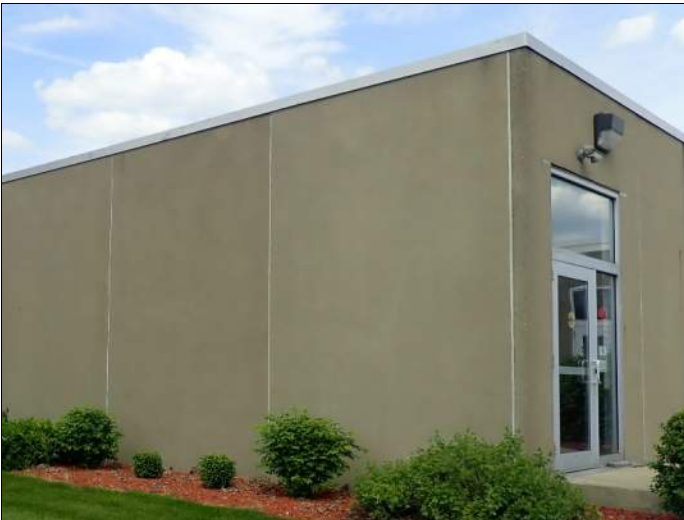
Typical precast concrete wall panels
