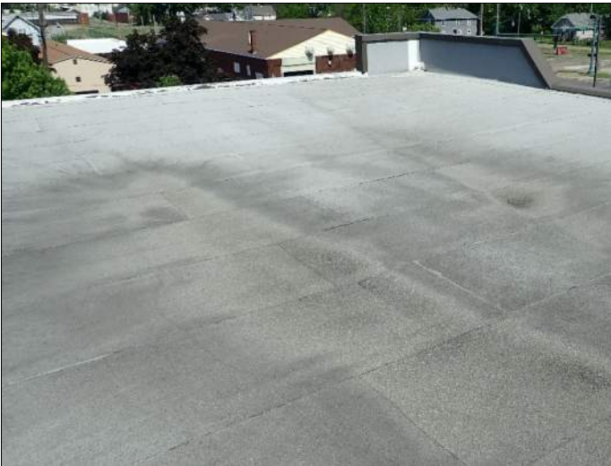
Modified bitumen membrane on upper roof
