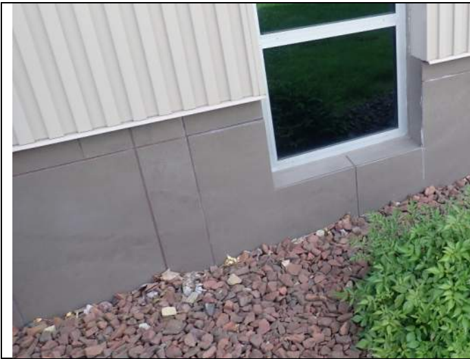
Exterior concrete tile wall finish
