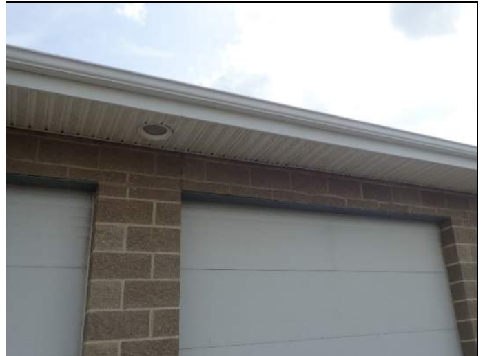
Outdoor recessed overhead lighting on garage
