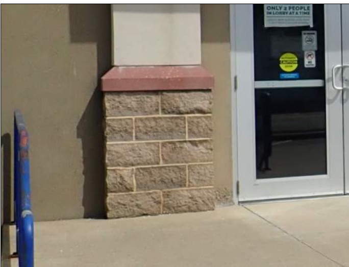
Exterior concrete masonry veneer
