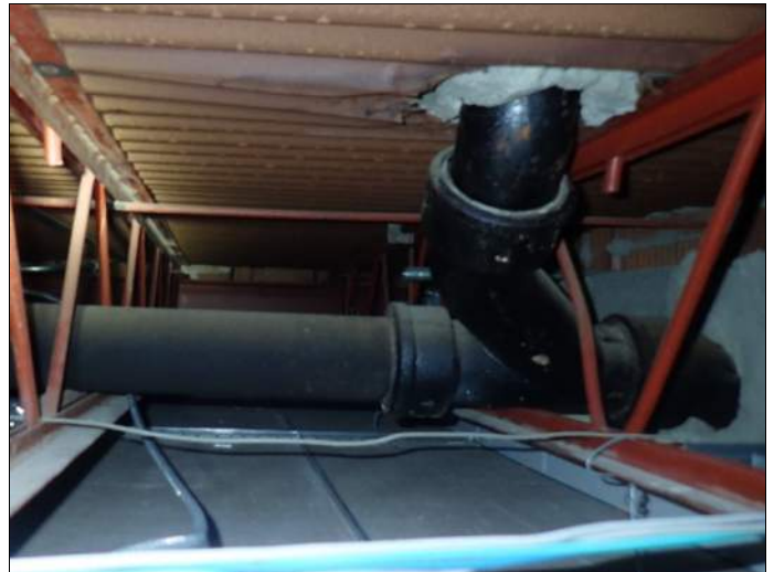
Filled metal deck floor on steel joists
