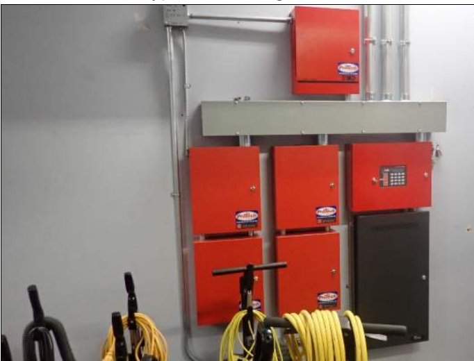
Fire alarm system control panel
