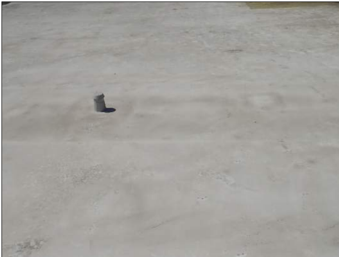
EPDM membrane on lower roof
